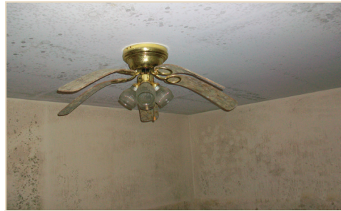
PHOTO 1 Mold growth caused by elevated relative humidity.
