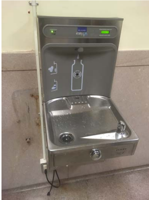
Photo 9 – 1 st Floor Hallway The compressor for the hydration station was making a very loud noise and was unplugged.
