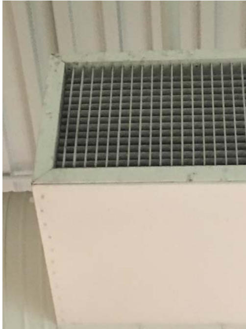
Photo 11– IMC Mold growth was observed on sections of the exposed duct work.
