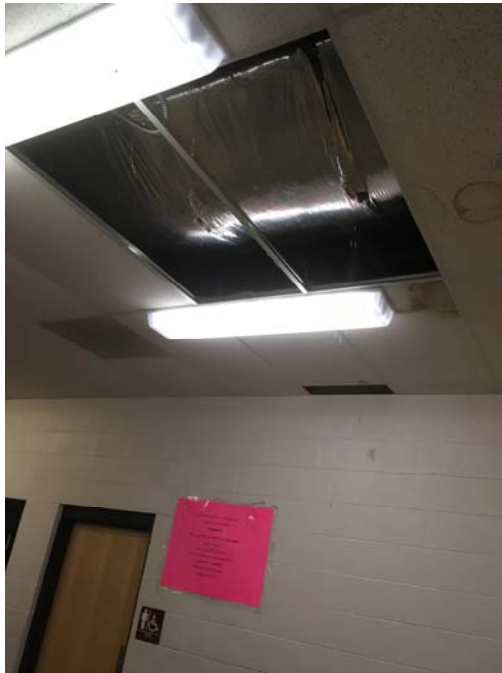
Photo 6 – Hallway outside Room 106 Condensate was leaking from a section of duct work located above the suspended ceiling.
