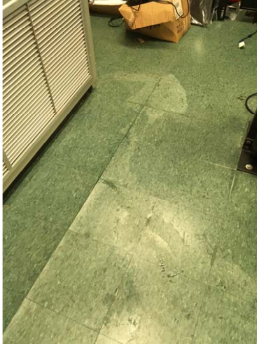
Photo 17 – IMC 134 MDF Room A delaminated section of floor tile was observed from the leaking condensate pump.
