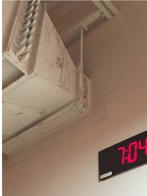
Photo 9 – IMC Mold growth was observed on sections of the exposed duct work.
