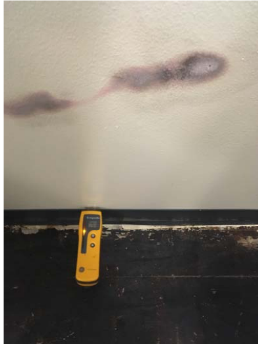
Photo 3 – Room 102 Mold growth was observed on the wallboard to the right of the unit ventilator.
