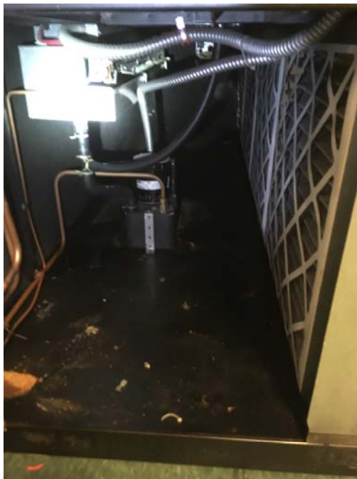
Photo 16 – IMC 134 MDF Room Water was leaking from the condensate pump.
