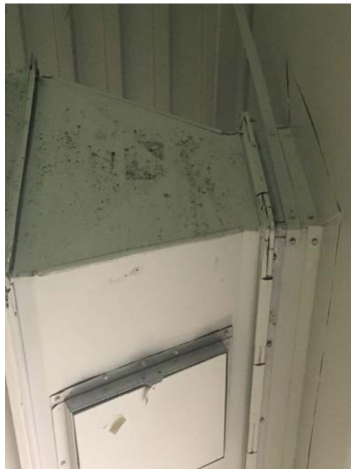
Photo 10 – IMC Mold growth was observed on sections of the exposed duct work.
