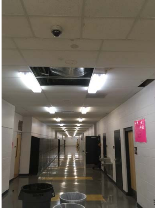
Photo 5 – Hallway outside Room 106 Condensate was leaking from a section of duct work located above the suspended ceiling.
