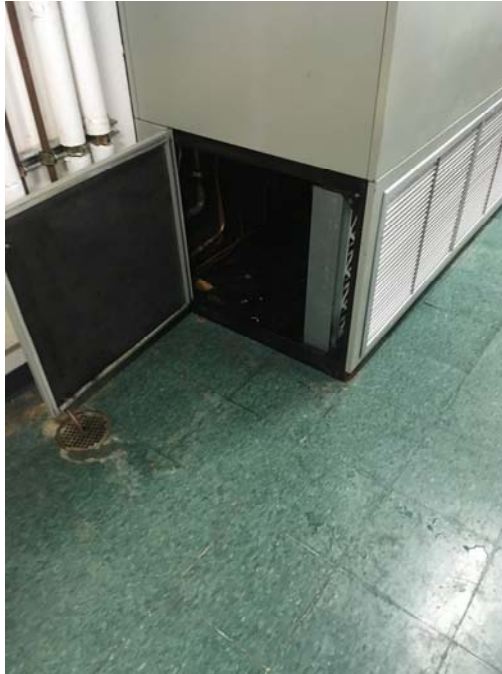
Photo 15 – IMC 134 MDF Room Water was leaking from the condensate pump.
