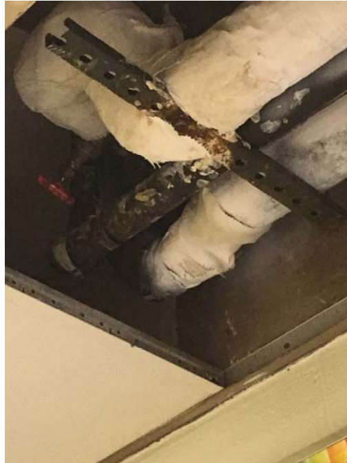
Photo 1 – Room 105 Condensation was leaking from the ceiling and a ceiling tile was missing.
