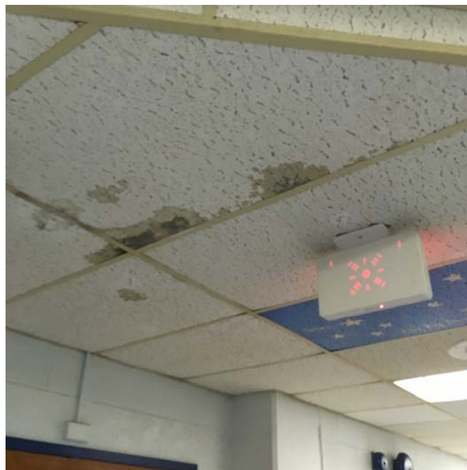
Photo 12 -Basement Hallway Water stained and moldy ceiling tiles were observed.
