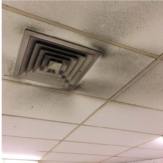
Photo 21 – Art Room 6 Particulate accumulation was observed on the supply diffuser and ceiling tiles.
