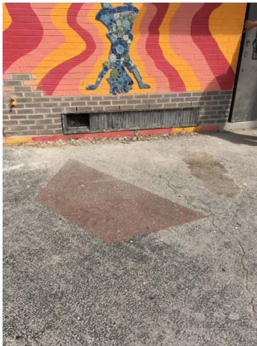
Photo 45- Exposed intake grille
