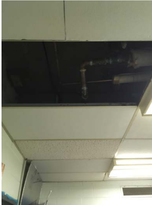
Photo 43- Practice Room A A missing ceiling was noted, no signs of active leaks were observed.
