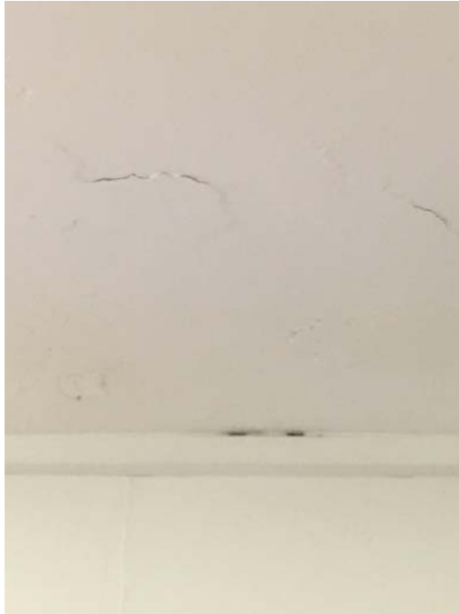
Photo 52- Room 210 Small delaminated sections of the concrete ceiling were observed.
