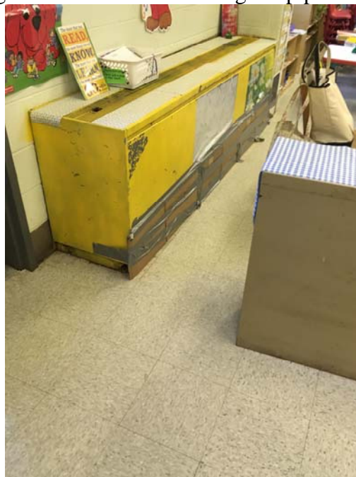
Photo 47- Room 1 The back of the cabinet is rotted allowing outdoor air into the room.
