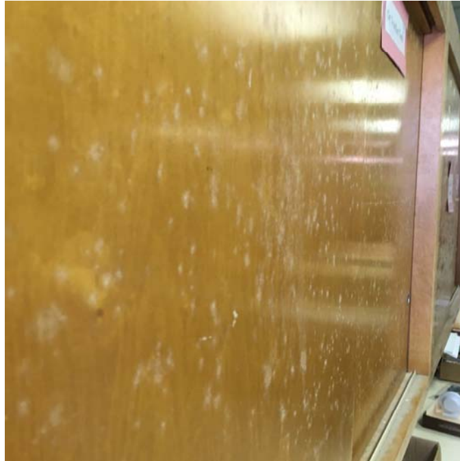
Photo 29 – Art Room 6 Mold growth was observed on the wooden cabinetry.
