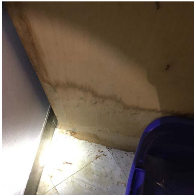
Photo 18 – Art Room 6 Mold growth was observed on the wooden cabinetry.
