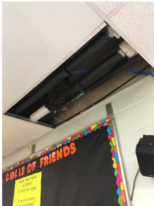
Photo 2 – Room 106 Condensation was leaking from the ceiling and a ceiling tile was missing.
