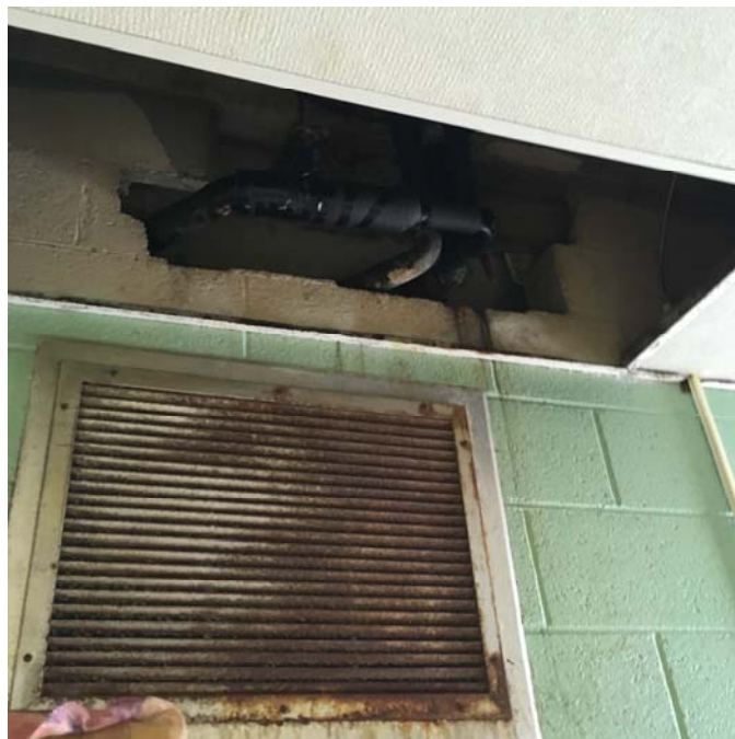
Photo 26 – Art Room 6 Condensation was leaking from the ceiling.
