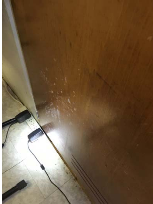
Photo 37 – Music Room 5 Mold growth was observed on the wooden cabinetry.
