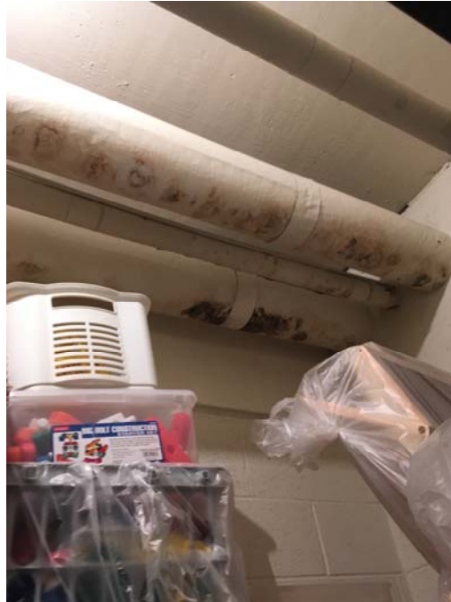
Photo 46- Room 1 closet Mold growth was observed fiberglass pipe insulation.
