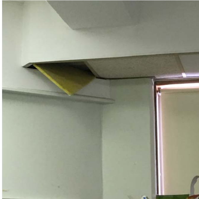
Photo 5 – Room 108 A ceiling tile fell in the corner.
