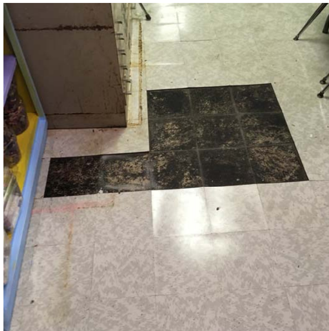
Photo 22 – Art Room 6 Delaminated 9"x9" floor tile was observed.
