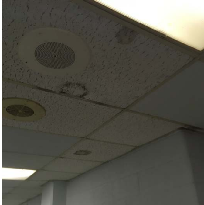
Photo 13 – Basement Hallway Water stained and moldy ceiling tiles were observed.
