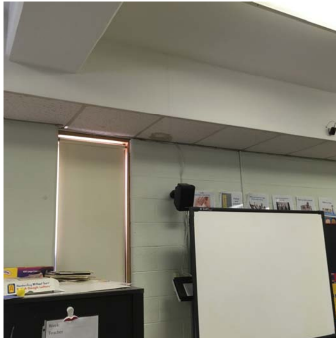
Photo 4 – Room 108 A water stained ceiling tile was observed.
