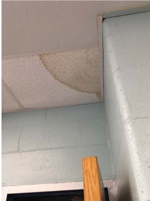
Photo 50- Room 211 A water stained ceiling tile was observed next to the closet.
