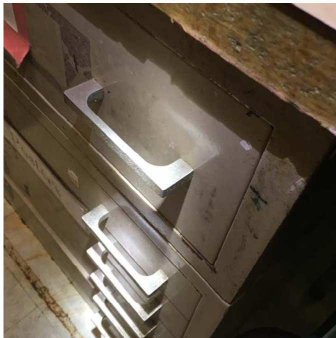
Photo 24 – Art Room 6 Mold growth was observed on the metal cabinetry.
