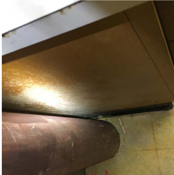
Photo 31 – Art Room 6 Mold growth was observed on the wooden cabinetry.
