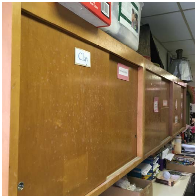
Photo 28 – Art Room 6 Mold growth was observed on the wooden cabinetry.
