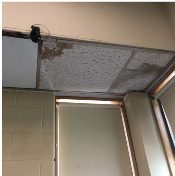
Photo 10 – Room 111 Water stained ceiling tiles were observed.
