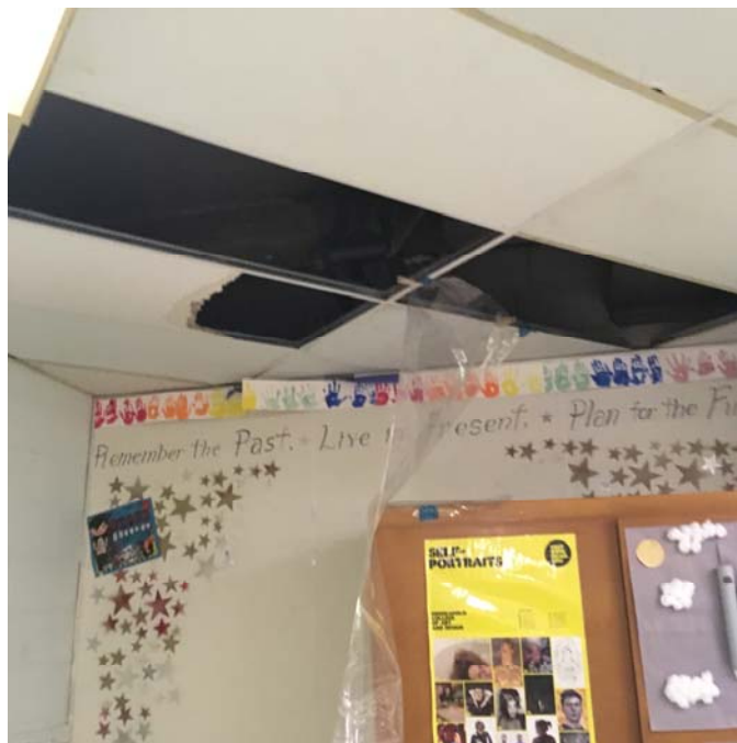
Photo 16 – Art Room 6 Condensation was leaking from the ceiling.
