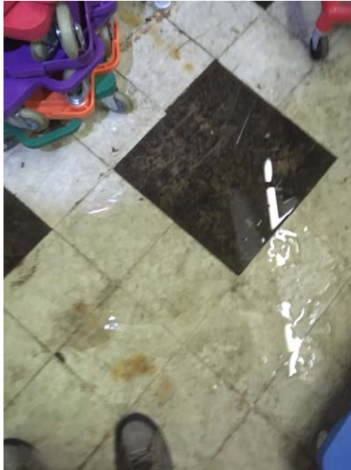
Photo 41- Music Suite Air Handler Room Standing water was observed on the floor and delaminated 9"x9" floor tile was observed.
