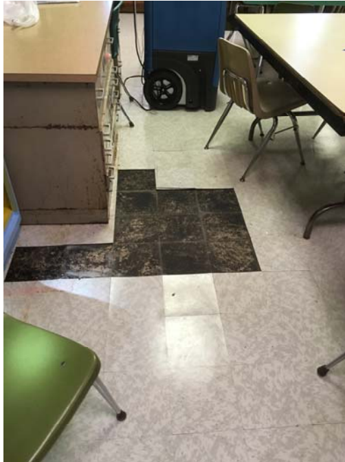
Photo 44- Art Room A section of delaminated floor tile was observed.
