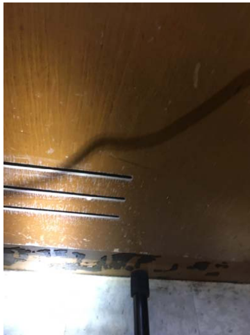
Photo 38 – Music Room 5 Mold growth was observed on the wooden cabinetry.
