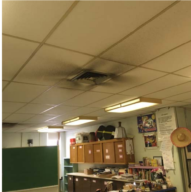
Photo 23 – Art Room 6 Particulate accumulation was observed on the supply diffusers and ceiling tiles.
