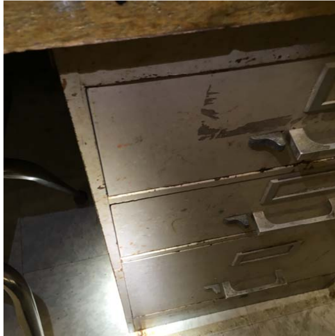
Photo 25 – Art Room 6 Mold growth was observed on the metal cabinetry.
