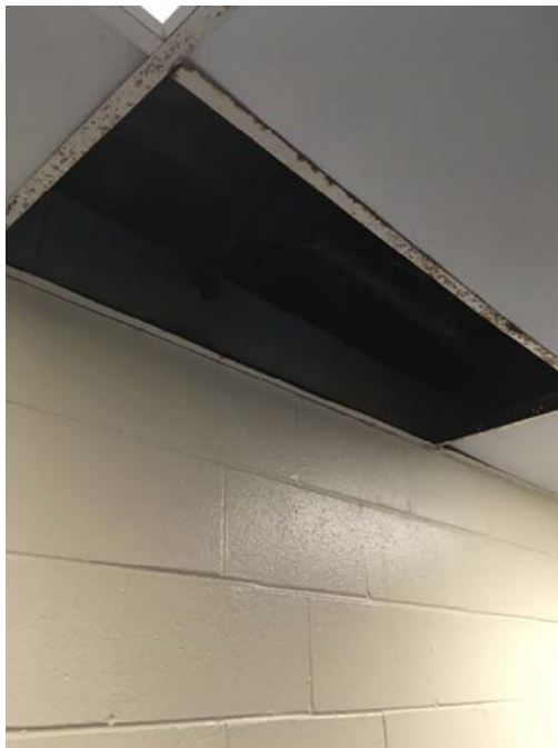
Photo 42- Gym Boy's Room A missing ceiling tile was observed and condensate appeared to be leaking from a pipe.
