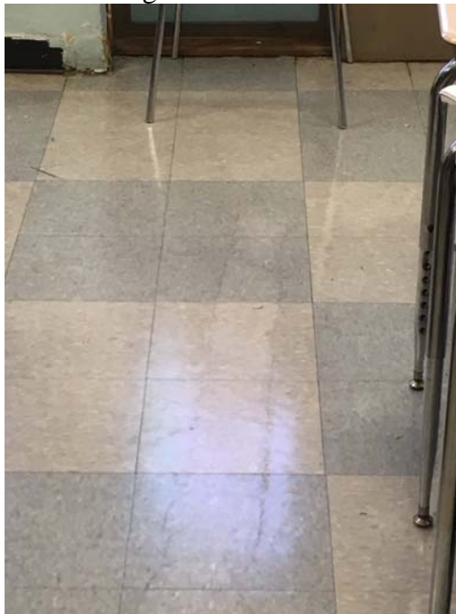
Photo 51- Room 211 A water stain trail appeared to be coming from the window. The occupant reported water intrusion on the floor during heavy rain.
