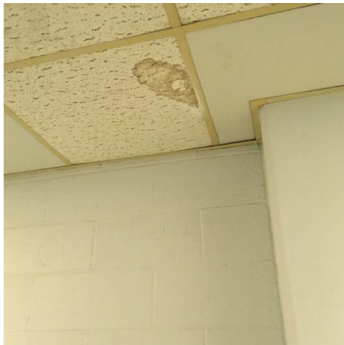
Photo 6 –Room 105 A water stained ceiling tile was observed.
