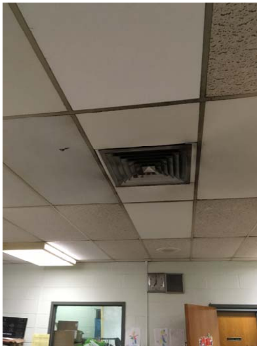
Photo 44- Instrumental Room Particulate accumulation was observed on the supply diffusers.
