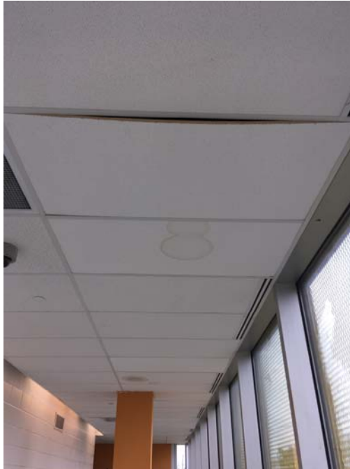
Photo 3 – 2 nd Floor Hallway (Race Street) Water stained ceiling tiles were observed.
