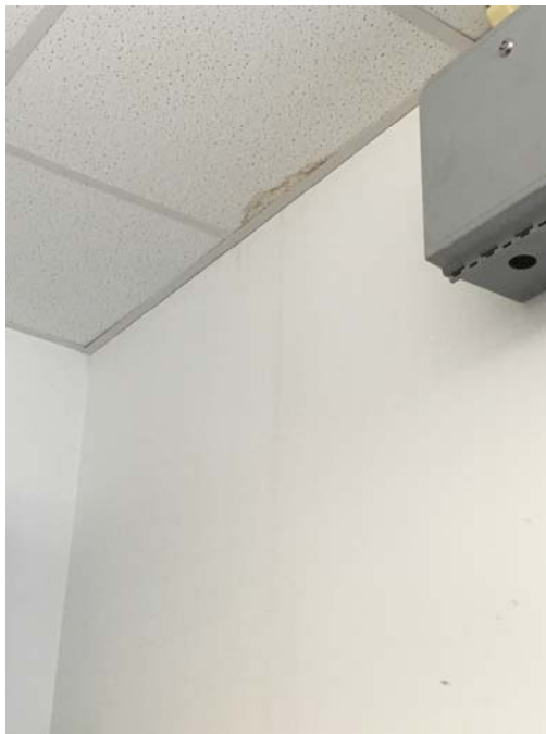
Photo 4 – Room 214 Water staining was observed on the ceiling tiles and wallboard.
