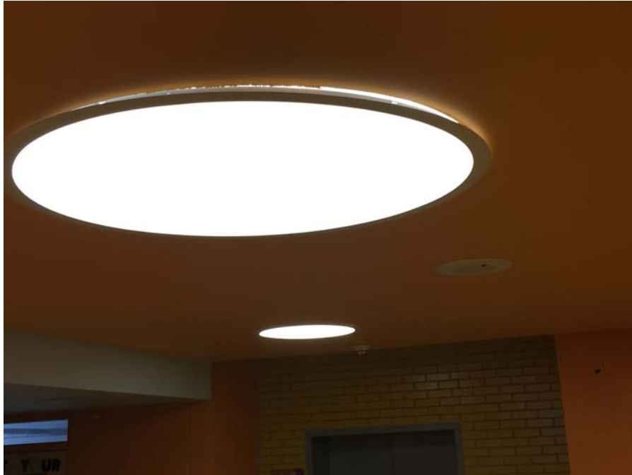
Photo 5 – 2 nd Floor Hallway The light trim was hanging below the ceiling.
