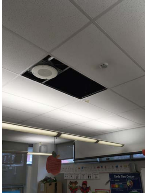
Photo 7 – Room 108 A missing ceiling tile was noted.
