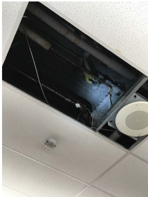
Photo 8 – Room 108 A water line was repaired; however, the lines need to be insulated.
