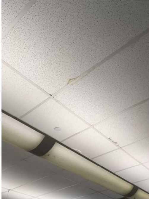
Photo 11– Room 109 A water stained ceiling tile was observed.
