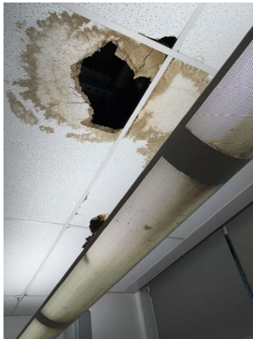
Photo 6 – Room 107 Water stained and missing ceiling tiles were observed.
