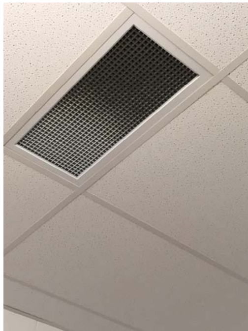
Photo 10 – Room 109 Particulate accumulation was observed on the relief grilles.
