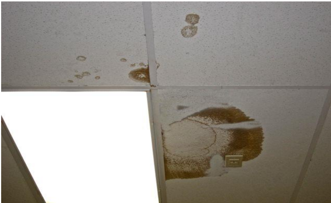
OEC Main Building - 12/2/13 - Library - 3 rd floor - Water damaged/stained ceiling tiles
