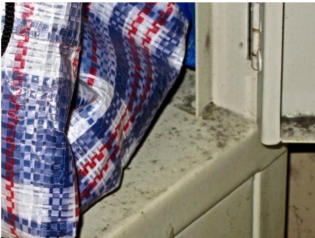
OEC Annex -12/2/13 - Classroom 1 - suspect mold growth in storage cabinet - close up
