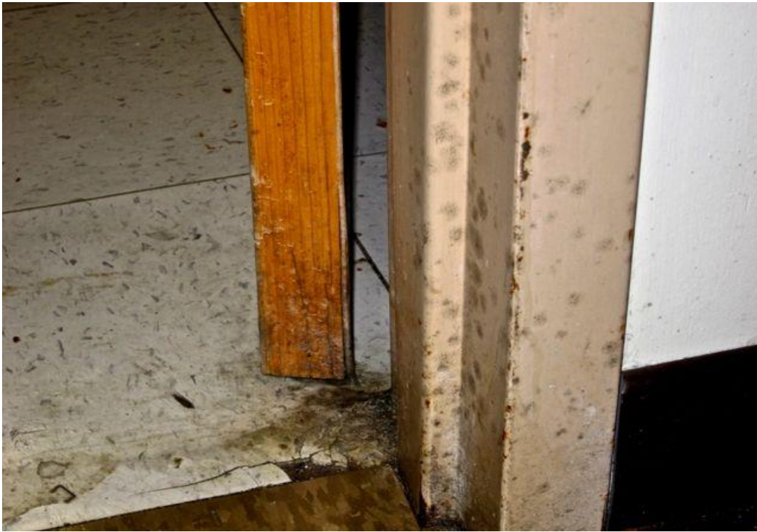
OEC Annex -12/2/13 - Classroom 1 - suspect mold growth on door frame
