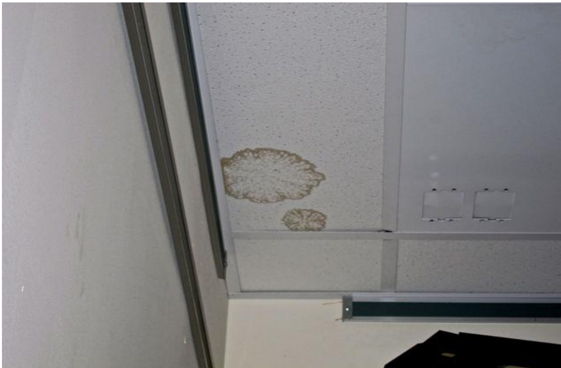
OEC Main Building - 12/2/13 - Library - 3 rd floor - water damaged ceiling tiles
