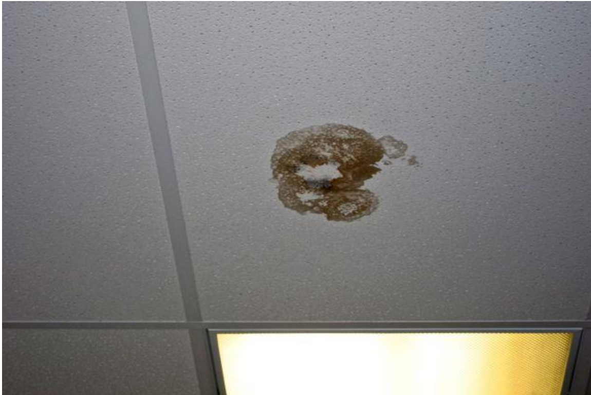
OEC Main Building - 12/2/13 - Library - 3 rd - Mold growth on ceiling tile
