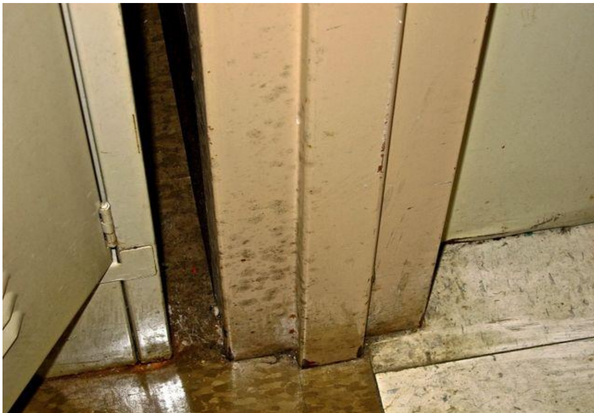
OEC Annex -12/2/13 - Classroom 23 - suspect mold growth on door frame
