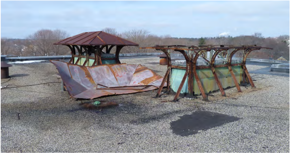
Ventilation hoods and close up detail of deteriorated pitch pocket where steel supports penetrate roof to fasten to underlying structure.
