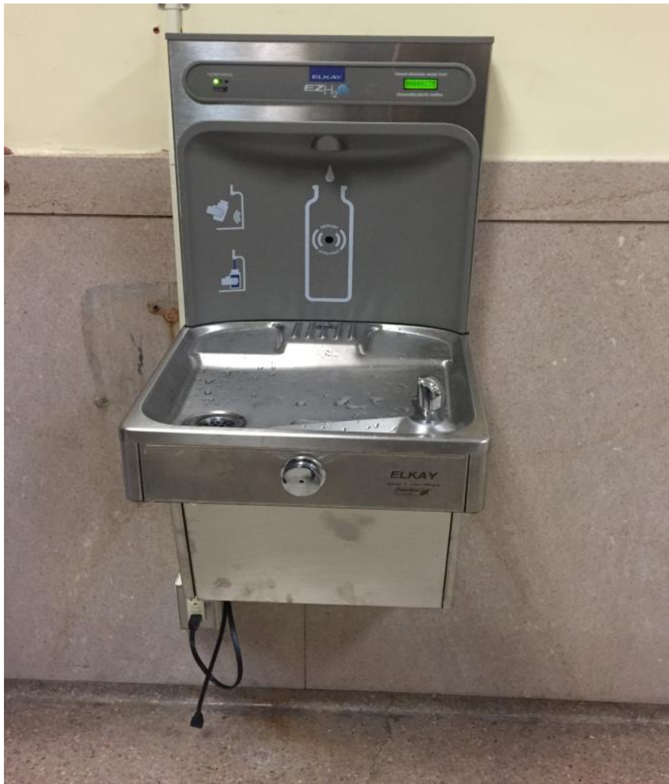
Photo 4 - Beeber MS - 12.13.2016 – 1 st Floor Hallway – Hydration Station – Bad Compressor & Unplugged
