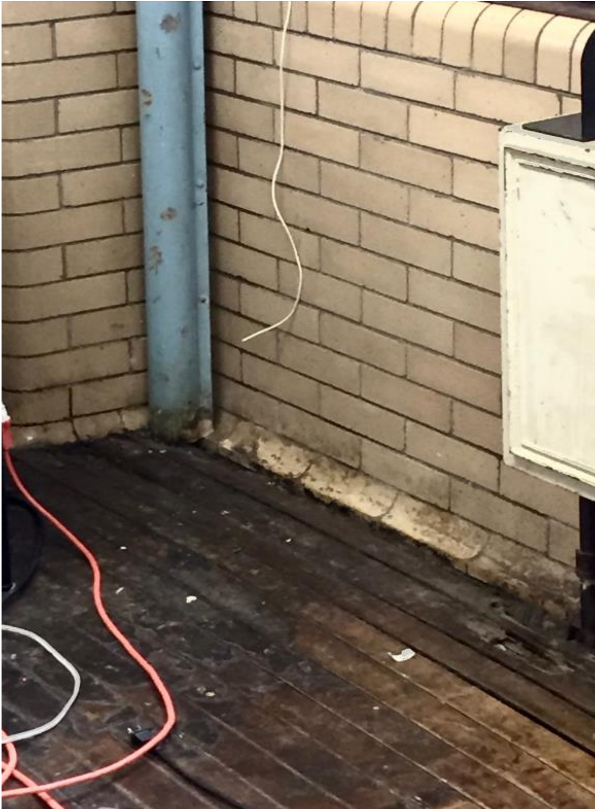
Photo 1 - Beeber MS - 12.13.2016 – Room 101 – Steam Leak at Radiator – Floor Damage
