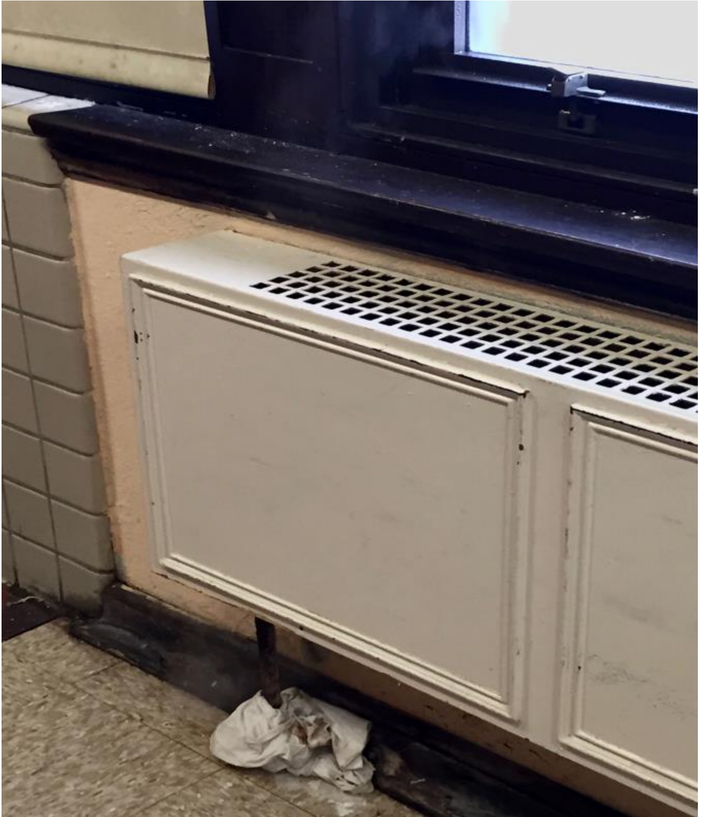
Photo 3 - Beeber MS - 12.13.2016 – Room 108 – Steam leak at radiator underneath floor – baseboard impacted
