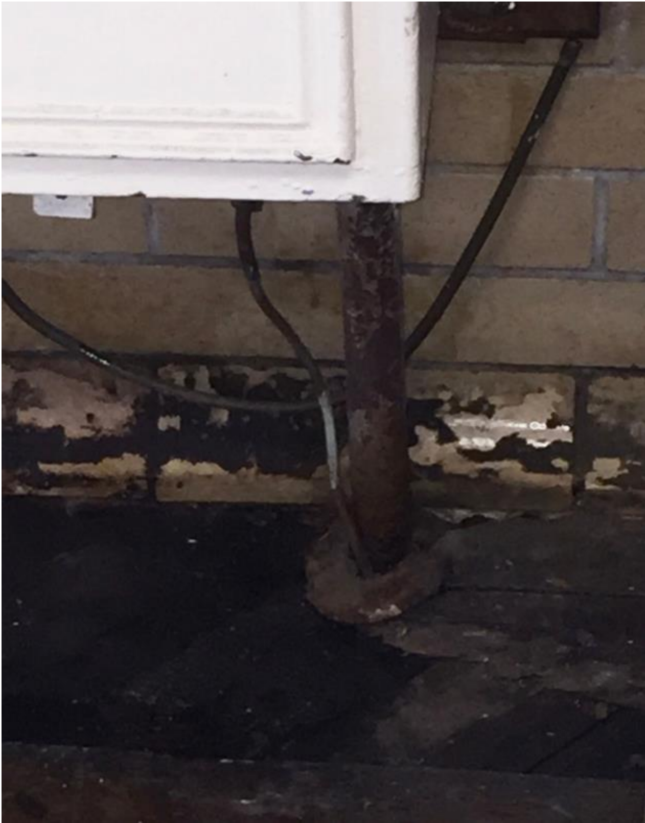
Photo 2 - Beeber MS - 12.13.2016 – Room 103 – Steam Leak at Radiator – Floor Damage
