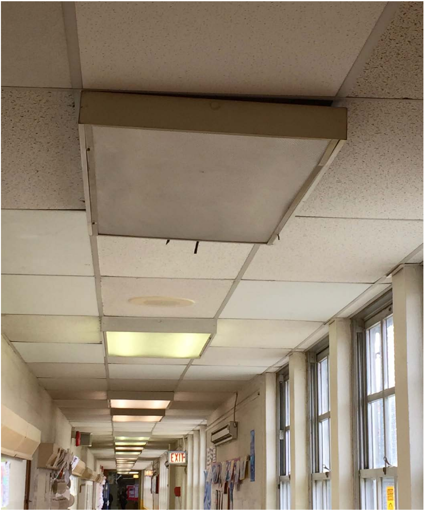
Photo 1 – Solis Cohen ES - 12.16.2016 – Main Office Hallway – Ceiling Mounted Light Fixture – Not Fully Secured
