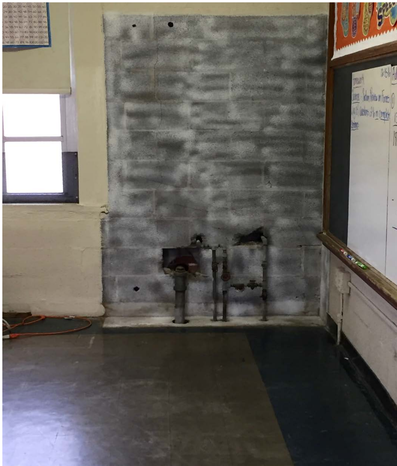
Photo 2 - Solis Cohen ES - 12.16.2016 – Room 29 – Condition after mold remediation and removal of impacted bookcase
