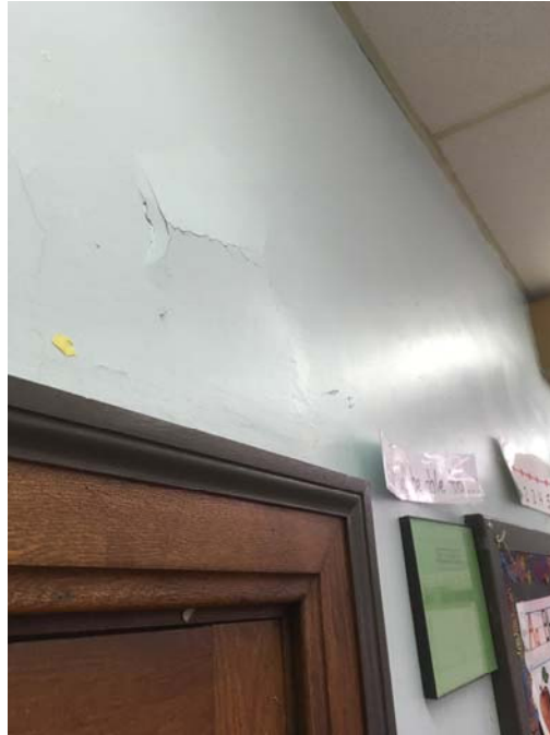
Photo 29 – Room 206 Delaminated sections of plaster wall were observed.
