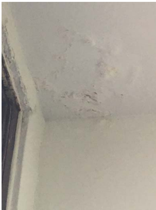
Photo 18 – 3 rd Floor Girl's Room Flaking paint and efflorescence was observed on the ceiling.
