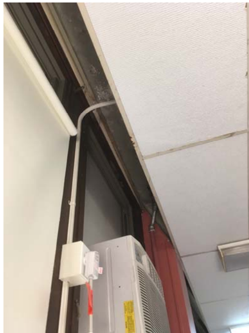
Photo 50 – Room 110 Missing ceiling tiles were observed above the windows.
