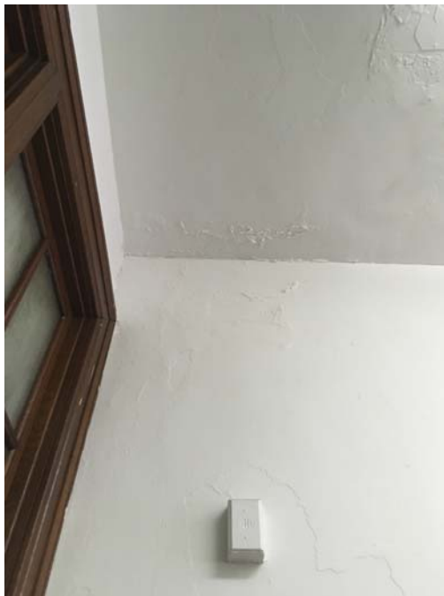
Photo 4 – 3 rd Floor Boy's Room Minor flaking paint and efflorescence was observed.
