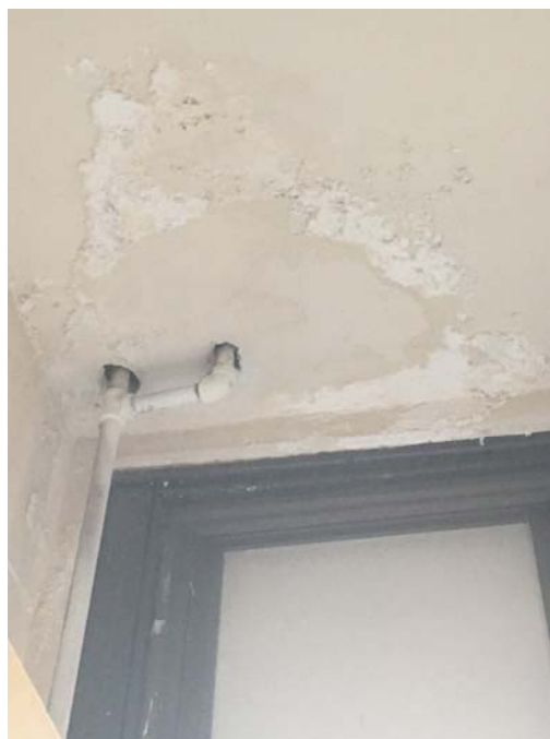
Photo 32 – Room 205 Closet Flaking paint and efflorescence was observed in this closet.
