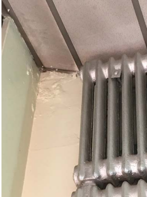
Photo 53 – Room 109 Kindergarten A minor section of efflorescence was observed nest to the wall mounted radiator.
