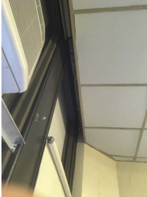
Photo 11– Room 304 A Minor flaking paint and efflorescence was observed above the window.
