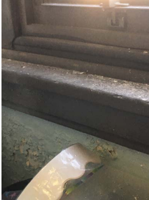
Photo 33 – Room 205 Closet Paint and plaster debris was observed on the window sill and floor.
