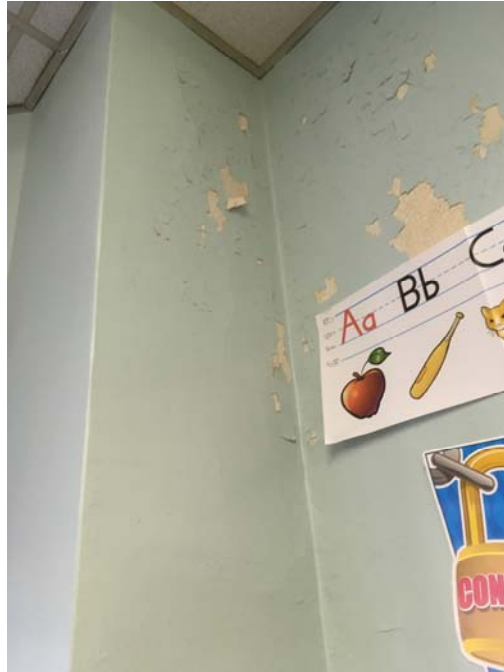
Photo 37 – Room 204 A Flaking paint was observed on the wall.
