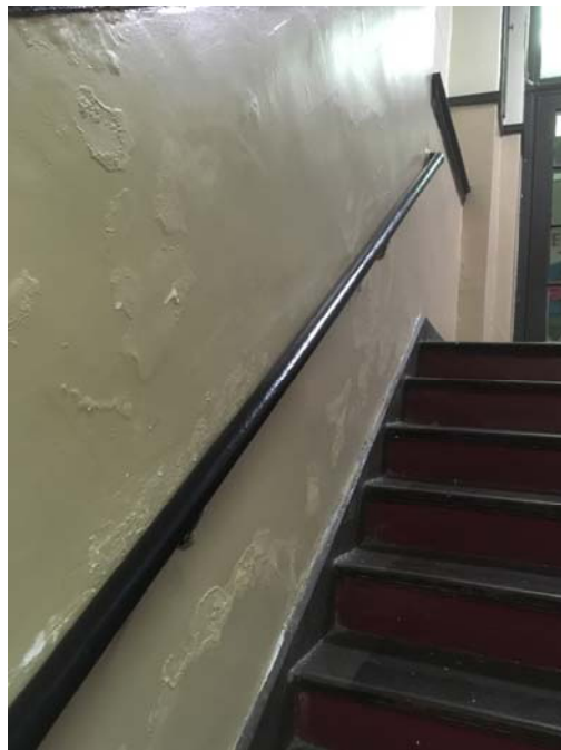
Photo 60 – Basement Boy's Stairwell to Gym This plaster wall was recently repaired, and is beginning to deteriorate again from moisture intrusion.
