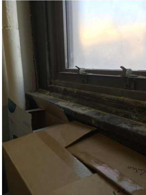
Photo 41 – Room 203 Closet Paint and plaster debris was observed on the window sill and floor.
