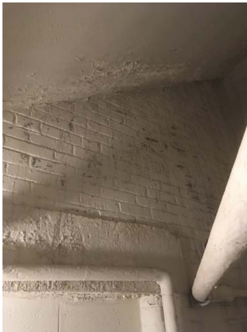
Photo 58 – Basement Boy's Side Custodial Closet Flaking paint and efflorescence was observed on the walls and ceiling.
