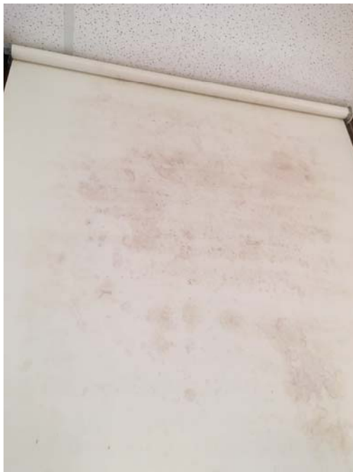
Photo 22 – IMC Suspect mold growth was observed on the shade over window #2.
