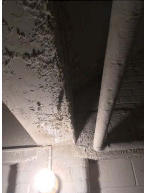
Photo 59 – Basement Boy's Side Custodial Closet Flaking paint and efflorescence was observed on the walls and ceiling.
