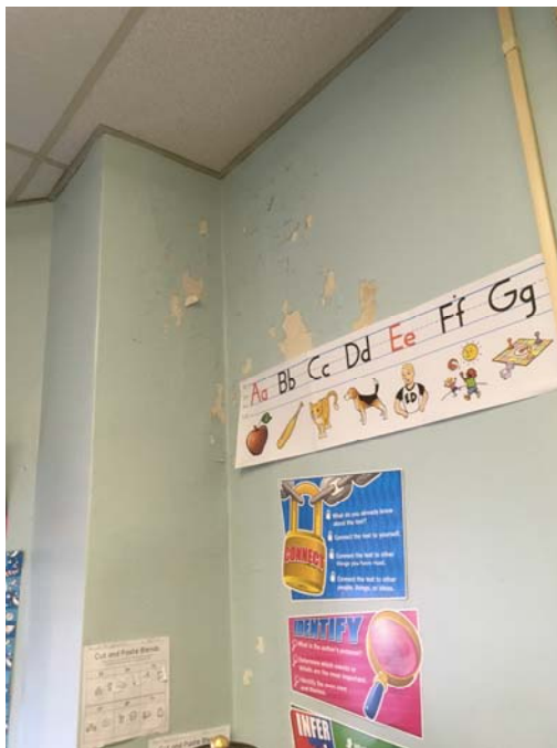
Photo 36 – Room 204 A Flaking paint was observed on the wall.
