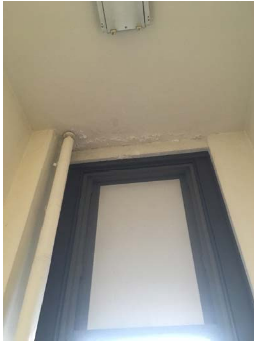
Photo 9 – Room 305 Closet Minor flaking paint and efflorescence was observed above the window.
