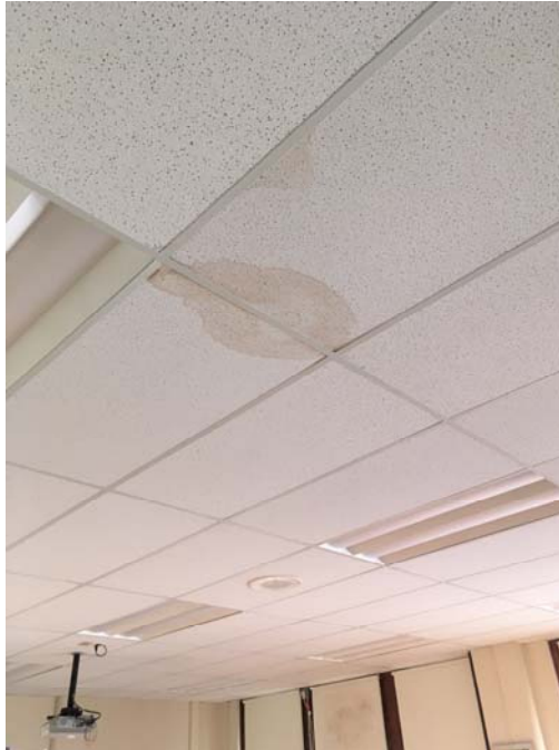
Photo 21 – IMC Water stained ceiling tiles were observed.
