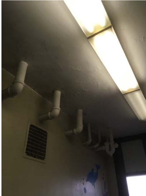
Photo 57 – 1 st Floor Boy's Room Flaking paint and efflorescence was observed on the ceiling.
