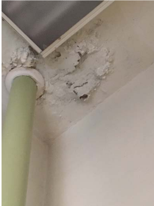
Photo 7 – Room 307 Closet Flaking paint and efflorescence was observed around the roof drain.
