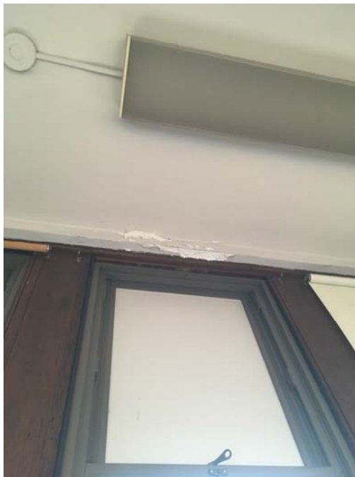
Photo 26 – Room 207 Closet Minor flaking paint and efflorescence was observed above the window.
