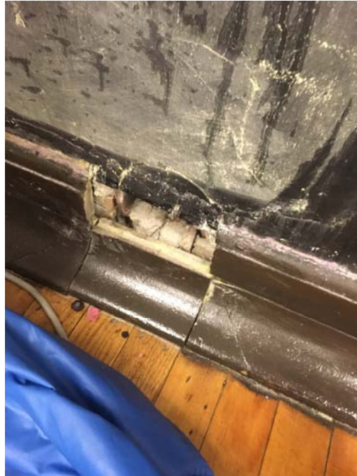
Photo 15 – Room 303 A small hole was observed on the baseboard on the back wall.
