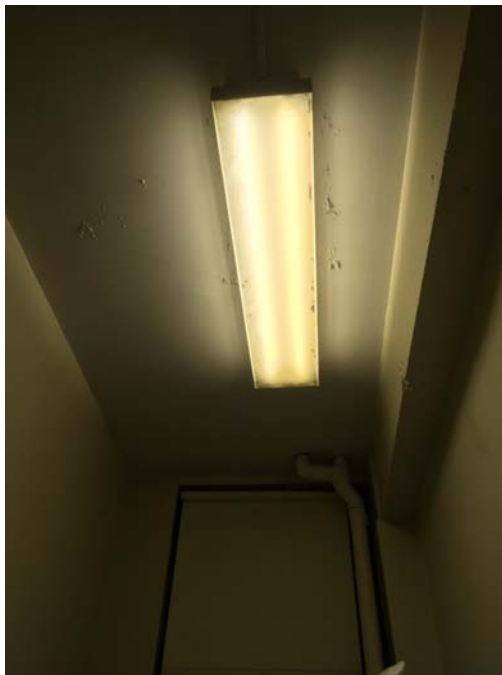
Photo 48 – Room 104 Closet Minor sections of flaking paint were observed on the ceiling.
