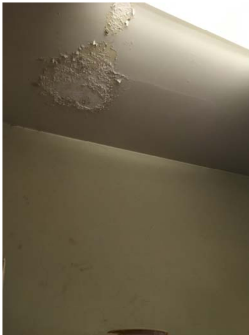
Photo 20 – Room 301 Closet Minor flaking paint and efflorescence was observed on the ceiling.
