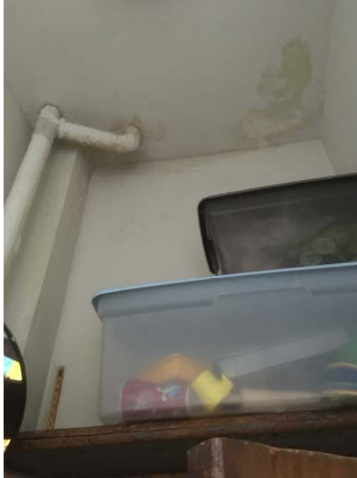
Photo 47 – Room 102 Closet Water stained was observed on the closet ceiling.
