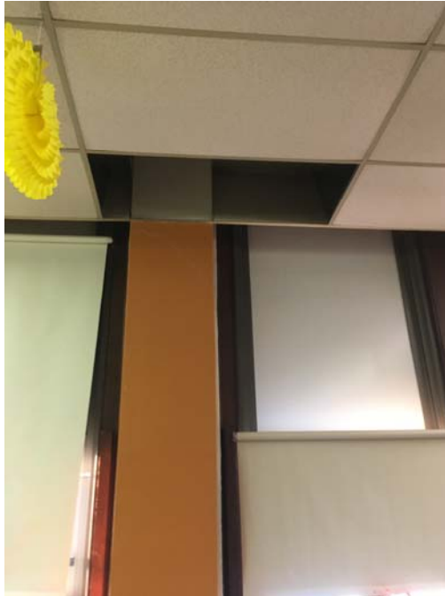
Photo 3 – Room 308 A missing ceiling tile was observed.
