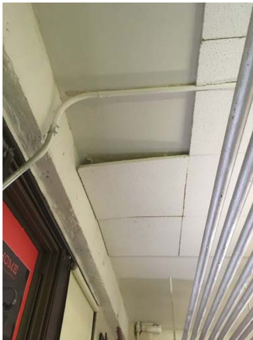
Photo 68 – Music Room A couple of delaminated ceiling tiles were observed.
