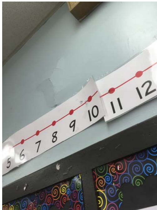
Photo 30 – Room 206 Delaminated sections of plaster wall were observed.
