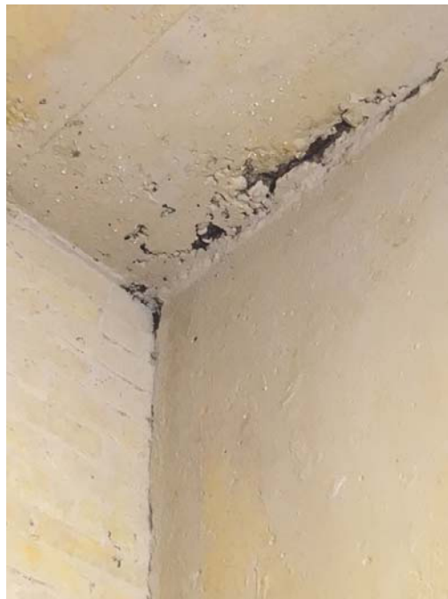
Photo 62 – Basement Boy's Side Stairwell Closet This closet had a strong musty odors and water droplets were observed on the ceiling.
