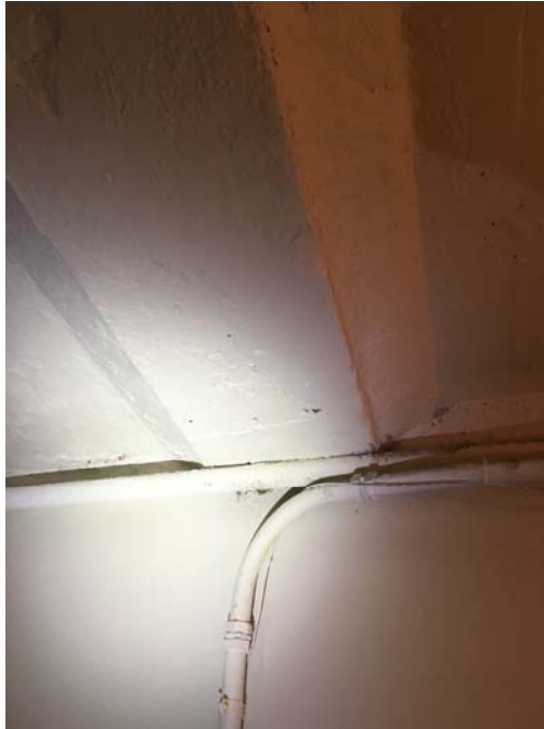
Photo 67 – Basement Girl's Side Stairwell Closet Water leaked from the ceiling during the heavy rain that occurred the night before the inspection.
