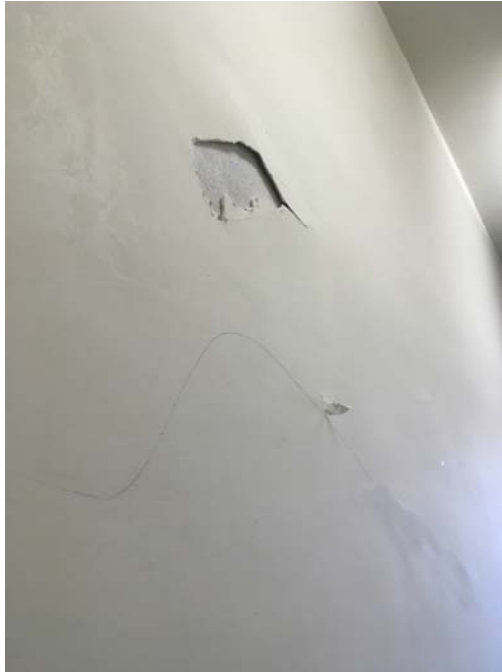
Photo 39 – Room 204 Closet A delaminated section of plaster wall was observed in this closet.
