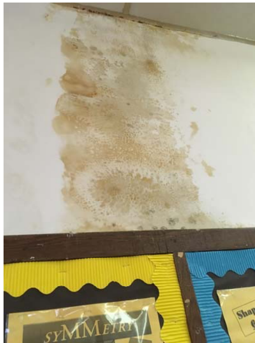
Photo 2 – Room 308 Mold growth was distributed over a moisture damaged section of plaster wall.
