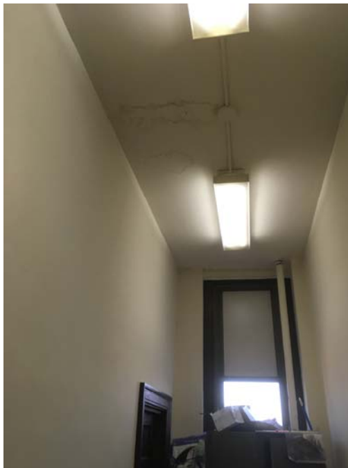
Photo 6 – Room 306 Closet Staining was observed on the plaster ceiling.
