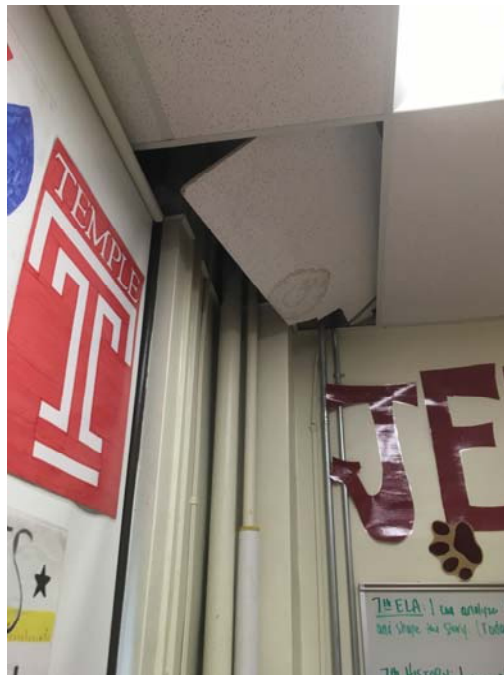
Photo 16 – Room 303 This ceiling tile was stained and about to fall from the suspended track.
