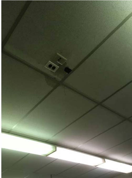
Photo 5 – Room 306 Water stained ceiling tiles were observed.
