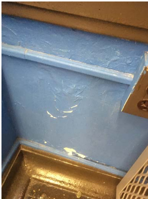
Photo 10 – Room 305 A minor section of damaged paint was observed below the window.
