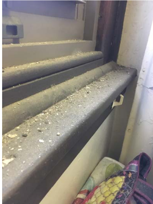
Photo 49 – Room 104 Closet Paint and plaster debris was observe don the window sill.
