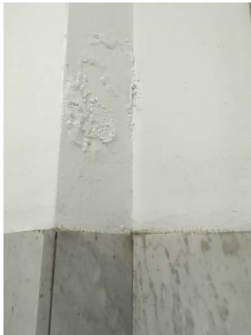
Photo 42 – 2 nd Floor Men's Room A minor amount of efflorescence was observed on the wall.
