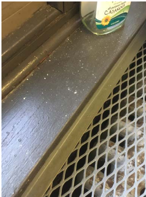
Photo 12 – Room 304 A A minimum amount of plaster debris was observed on the window sill.
