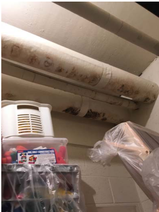
Room 3 Closet – Mold growth on fiberglass pipe insulation
