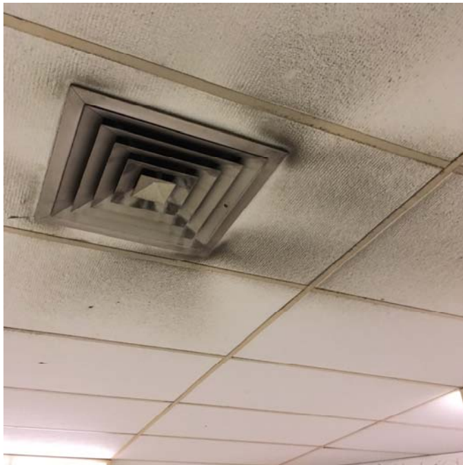
Photo 8 – Art Room 6 Particulate accumulation was observed on the supply diffuser and ceiling tiles.
