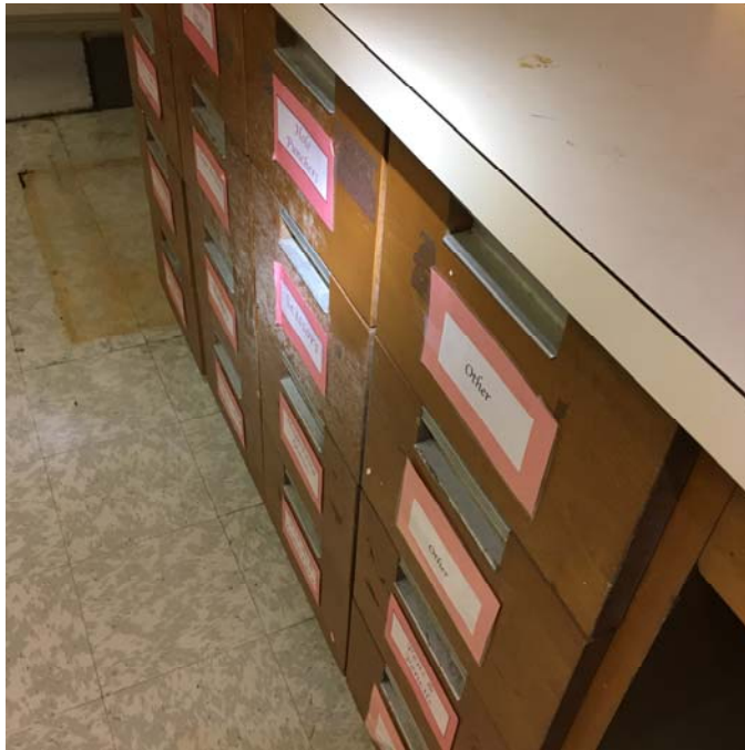
Photo 19 – Art Room 6 Mold growth was observed on the wooden cabinetry.
