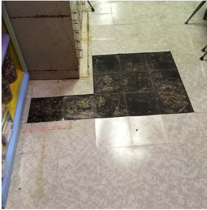
Photo 9 – Art Room 6 Delaminated 9"x9" floor tile was observed.
