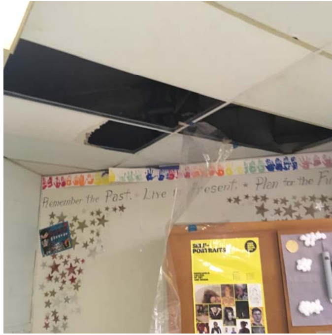
Photo 3 – Art Room 6 Condensation was leaking from the ceiling.
