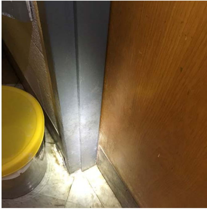
Photo 7 – Art Room 6 Mold growth was observed on the wooden doors and metal frames.
