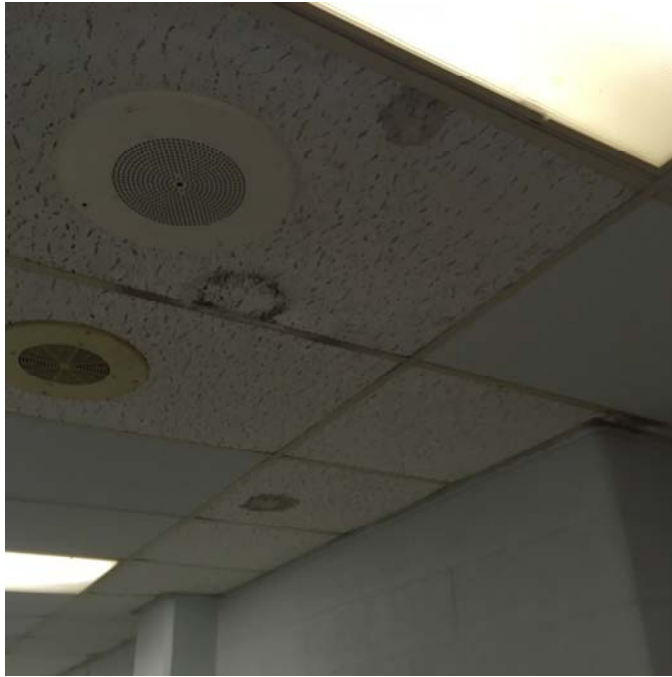
Photo 27 – Basement Hallway Water stained and moldy ceiling tiles were observed.
