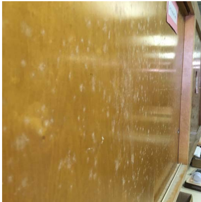
Photo 16 – Art Room 6 Mold growth was observed on the wooden cabinetry.
