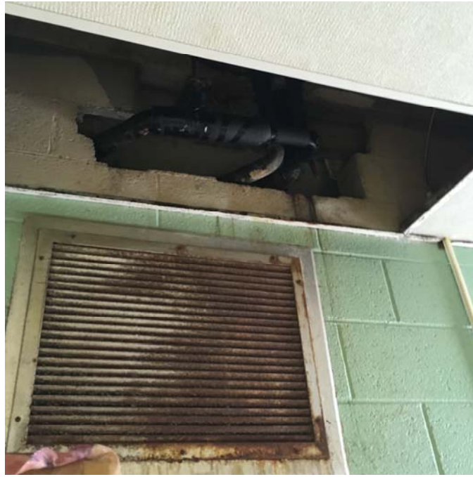
Photo 13 – Art Room 6 Condensation was leaking from the ceiling.
