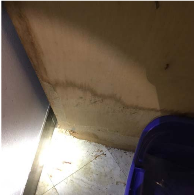
Photo 5 – Art Room 6 Mold growth was observed on the wooden cabinetry.
