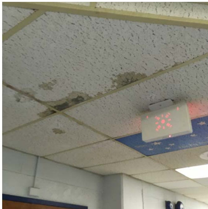
Photo 26 –Basement Hallway Water stained and moldy ceiling tiles were observed.
