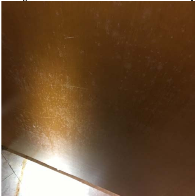
Photo 6 – Art Room 6 Mold growth was observed on the wooden cabinetry.
