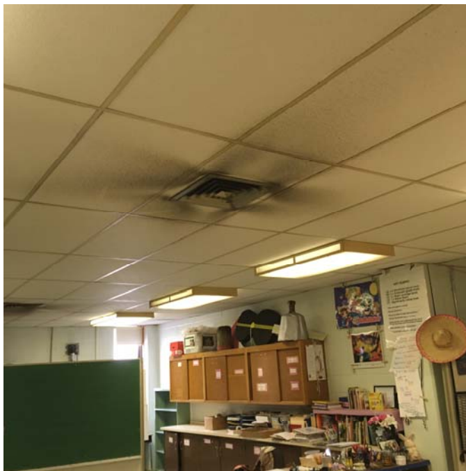
Photo 10 – Art Room 6 Particulate accumulation was observed on the supply diffusers and ceiling tiles.
