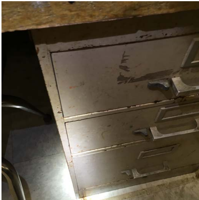
Photo 12 – Art Room 6 Mold growth was observed on the metal cabinetry.
