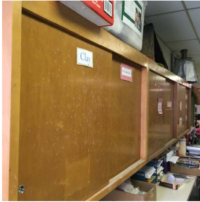
Photo 15 – Art Room 6 Mold growth was observed on the wooden cabinetry.
