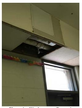
Photo 4 – Kindergarten Room 1 A missing ceiling tile and condensate was dripping from the ceiling. Wet fiberglass pipe insulation was observed above the suspended ceiling.
