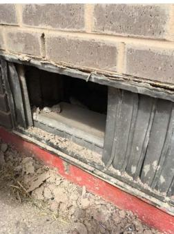
Photo 35 – Kindergarten Room 3 Outdoor air intake open to the interior from construction activity.
