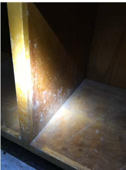
Photo 21 – Kindergarten Room 2 Mold growth was observed on the built-in wooden cabinetry and coat cubby.
