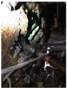
Photo 41 – Kindergarten Room 3 The condensate drip pan was missing. Condensate was dripping on the floor.
