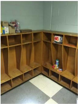
Photo 19 – Kindergarten Room 2 Mold growth was observed on the built-in wooden cabinetry and coat cubby.
