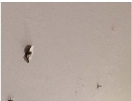
Photo 3 – Kindergarten Room 1 Small sections of spalling concrete ceiling were observed on the ceiling.
