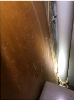
Photo 11– Kindergarten Room 1 Mold growth was observed on the wooden built-in cabinetry and coat cubby.
