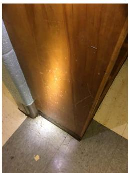
Photo 18 – Kindergarten Room 2 Mold growth was observed on the built-in wooden cabinetry and coat cubby.
