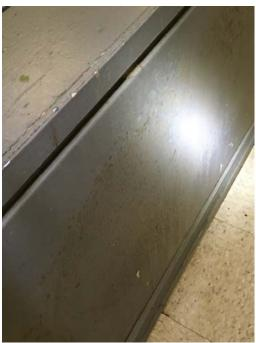
Photo 5 – Kindergarten Room 1 Mold growth was observed on the unit ventilator.
