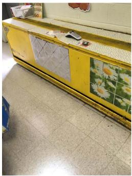
Photo 34 – Kindergarten Room 3 The return air tray was not seated properly and no air filters were observed inside this unit.
