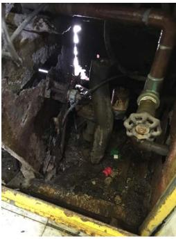
Photo 39 – Kindergarten Room 3 Daylight visible through the back of the unit ventilator.
