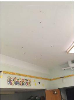
Photo 2 – Kindergarten Room 1 Small sections of spalling concrete ceiling were observed on the ceiling.
