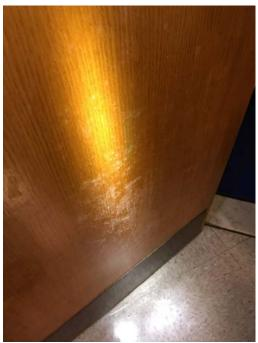
Photo 8 – Kindergarten Room 1 Mold growth was observed on the wooden door and metal frame.
