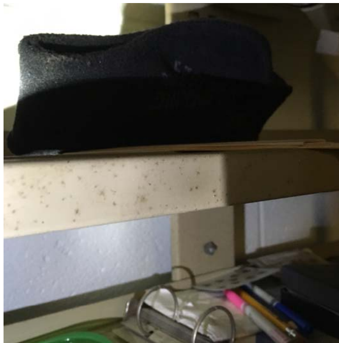
Photo 34 – Kitchen Staff Area Mold growth was observed on the coat rack.
