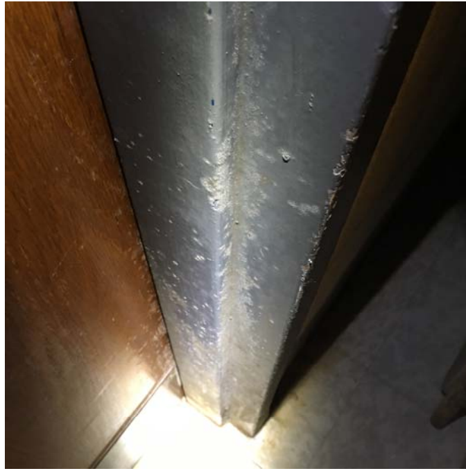
Photo 21 – Stage Mold growth was observed on the wooden door and metal door frame.
