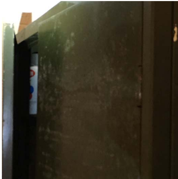
Photo 30 – Small Teacher's Storage Room Mold growth was observed on the metal storage units.
