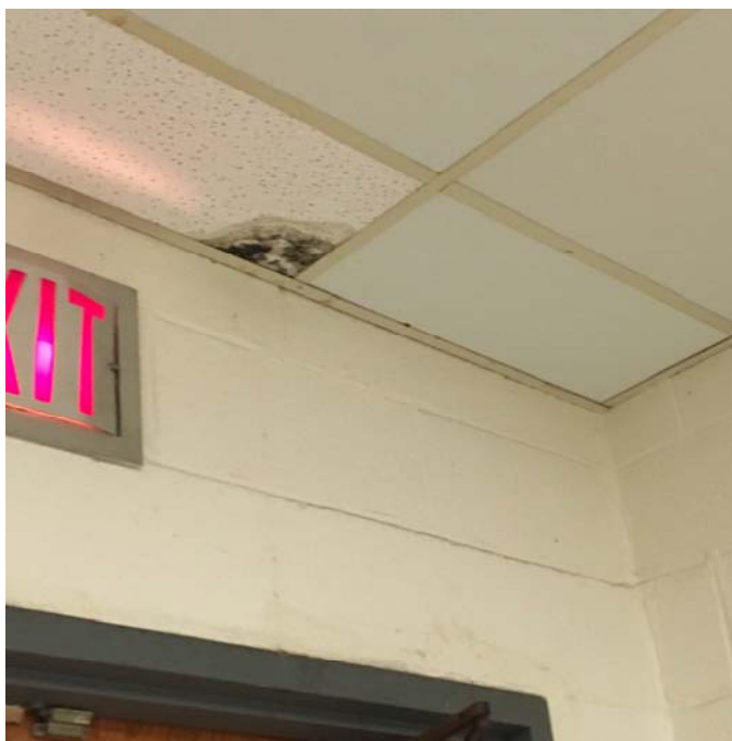
Photo 16 – Cafeteria A mold ceiling was observed by the 2 nd grade exit door.
