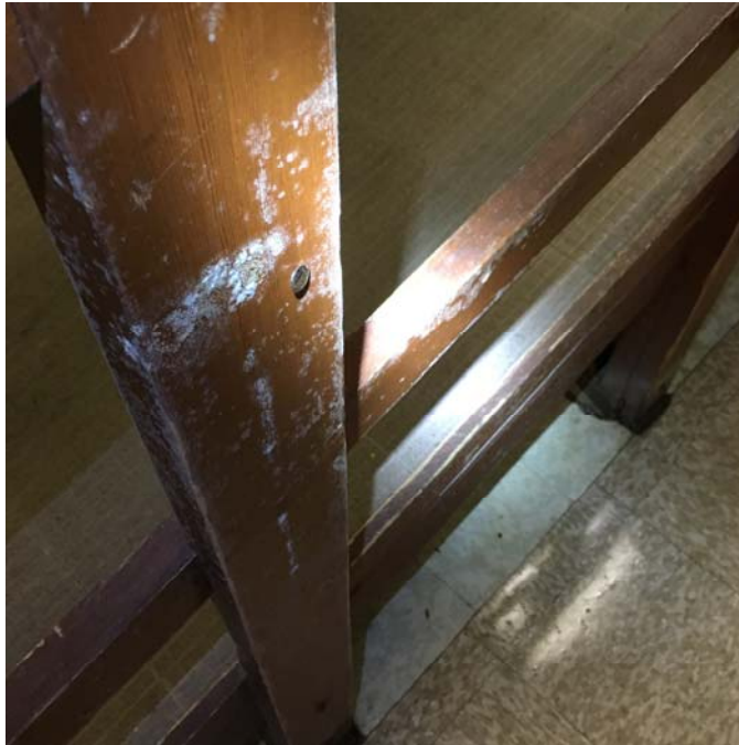
Photo 11– Cafeteria Mold growth was observed on the handicap ramp.
