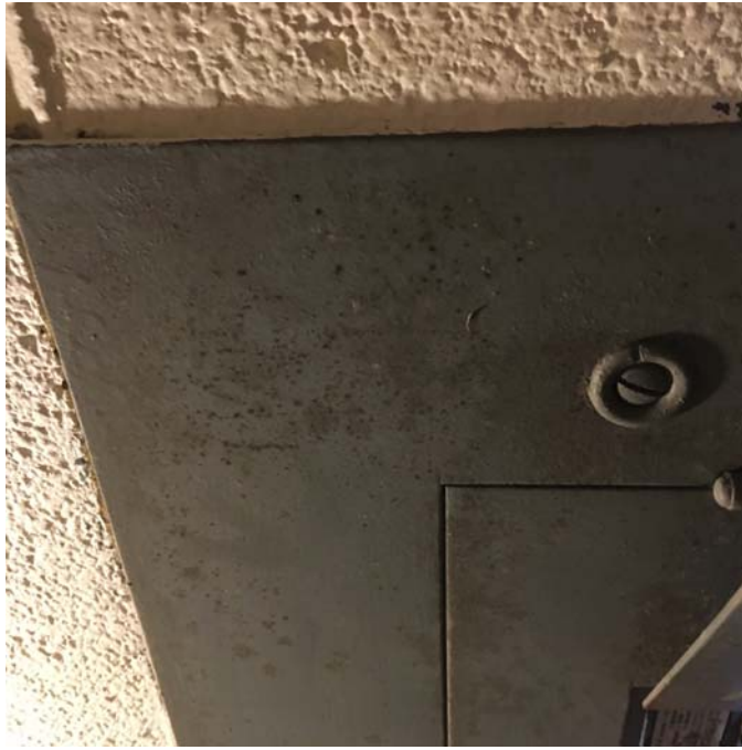
Photo 17 – Stage Mold growth was observed on the electrical panel covers.
