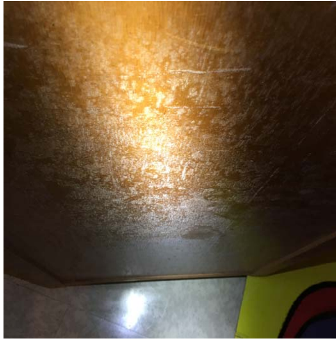
Photo 19 – Stage Mold growth was observed on the podium.
