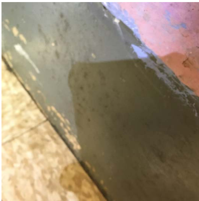
Photo 15 – Cafeteria Mold was observed on sections of the lower cinder block walls.
