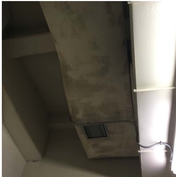
Photo 28 – Small Teacher's Storage Room Mold growth was observed on the fiberglass duct insulation.
